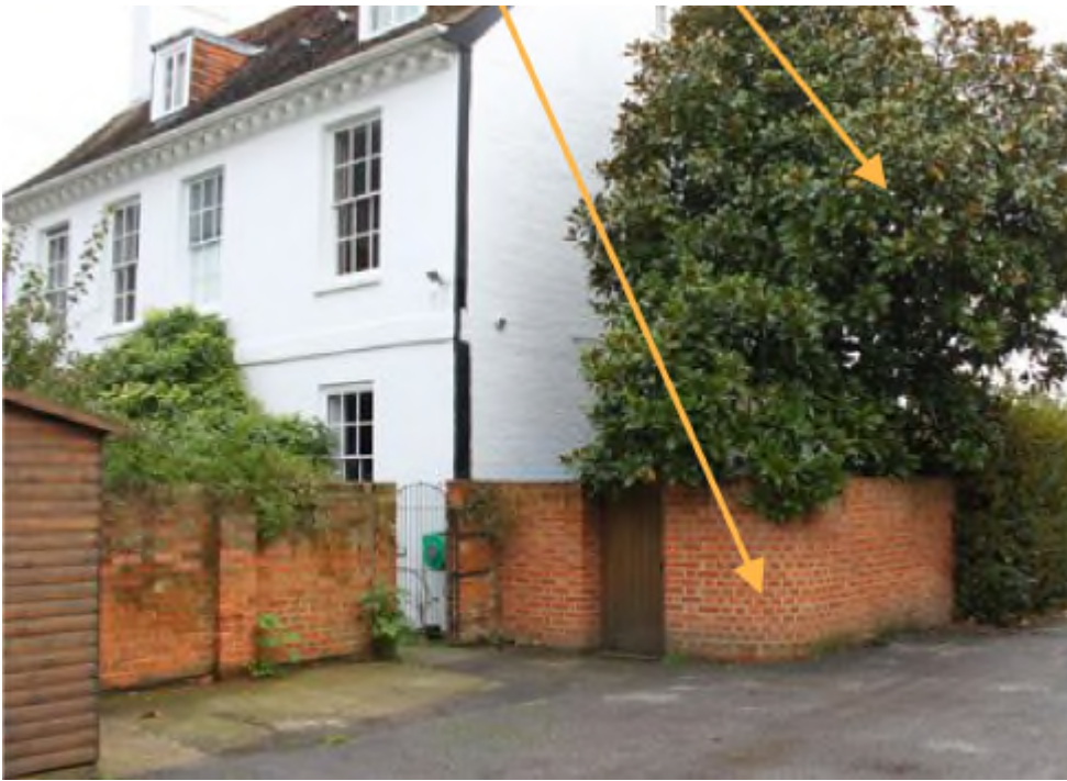
Figure 4. Shows the original southern wall (left of the photograph) – buttressed and Flemish Bond. Note, the contemporary wall to the right copies the style, but is obviously modern.
